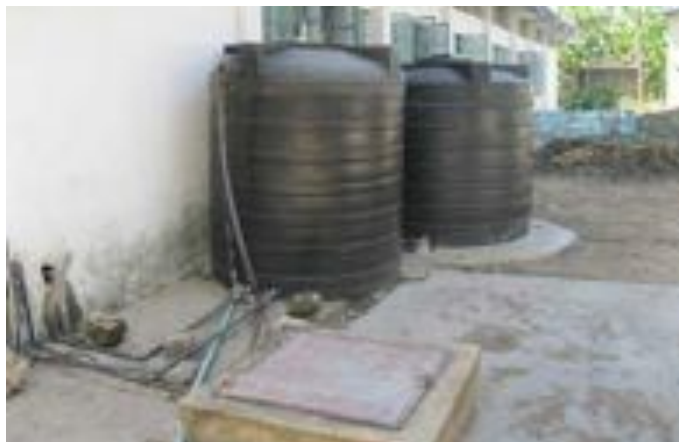
Tanks for water storage
